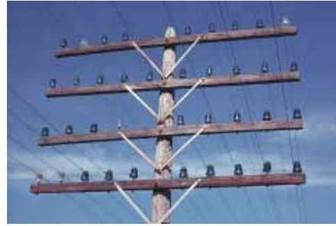
Electrical insulators on telephone poles are often made of glass because of its low electrical conductivity.
