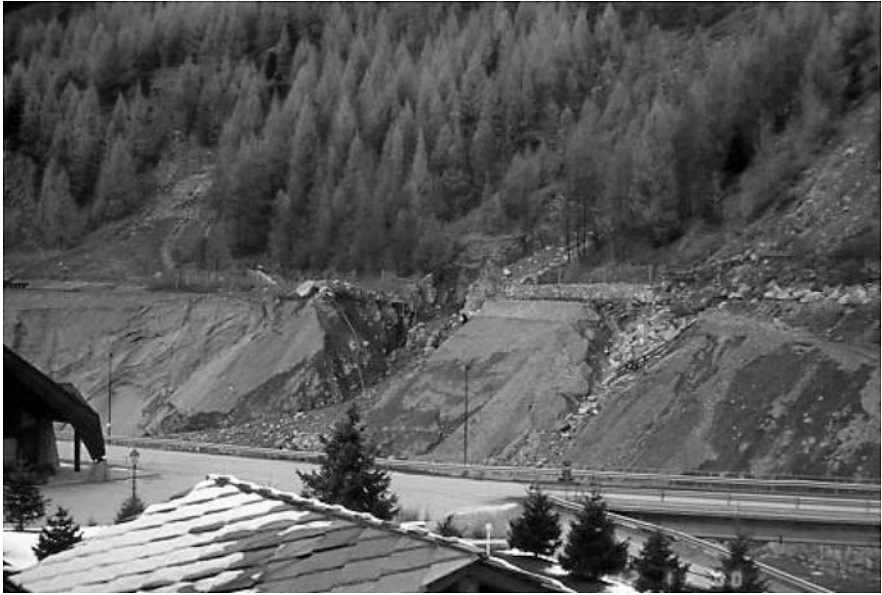
Fig. 5 Mining dump of magnetite overburden, periodically undergoing water erosion processes under intense autumn rain. Chromium oxides, sulphides and sulphates, heavy metals and trace elements slowly flow into the river below. (1,500 m a.s.l., Western Italian Alps) (Photo by F. Previtali)
