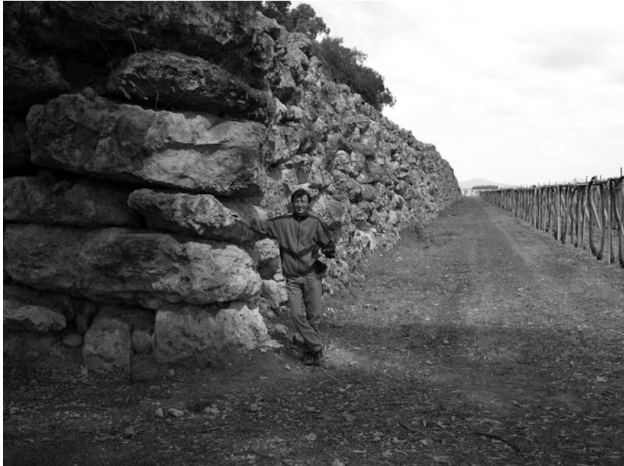
Fig. 3 Blocks of calccrete horizons removed in Sella e Mosca’s vineyard farm and piled up in the form of a “cyclopic” wall
