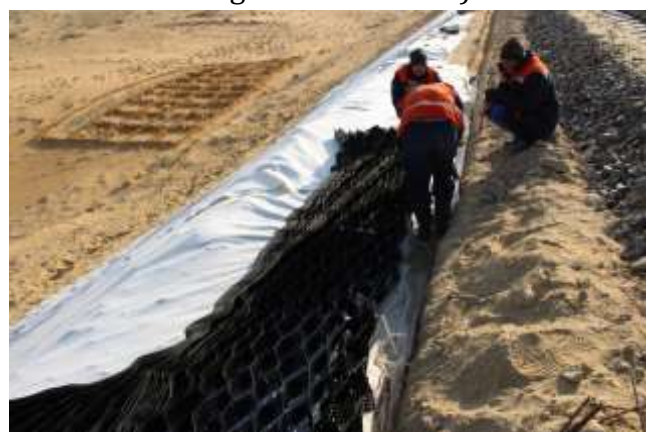
Figure-2. The process of installation of geogrids on the slopes of the subgrade (Kiyikli – Khizirbobo stage km 4199 PK 1)
