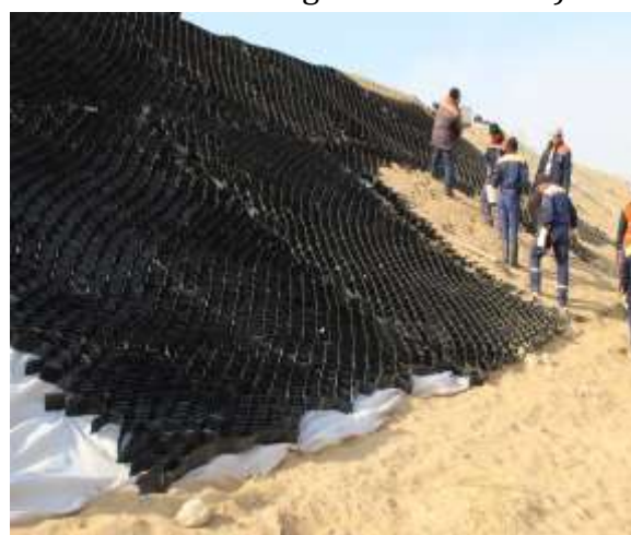
Figure-3. The process of filling the geogrid cells with local soil with parallel sowing of sand-loving grass seeds (Kiyikli – Khizirbobo stage km 4199 PK 1)
