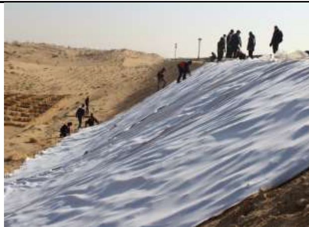
Figure-1. The process of laying geotextile on the slopes of the subgrade (Kiyikli – Khizirbobo stage km 4199 PK 1)
