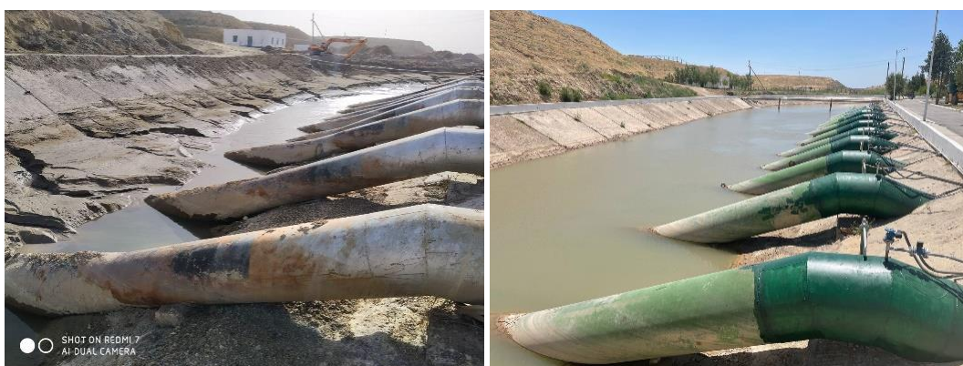
Figure 2. Reconstruction of suction pipelines (2022 compared to 2020) and cleaning of the water intake of the PS "Kiziltepa-1"
