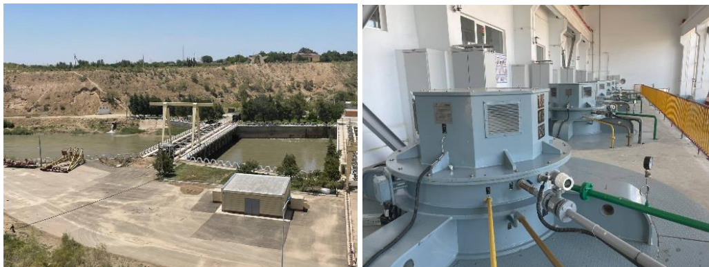
Figure 1. Reconstruction of the fore chamber of the hydroelectric complex of the PS "Kiziltepa" and the engine room of the PS "Kuyumazor" with new Chinese equipment
