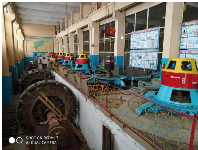
FIGURE 2. Modernization of pumps on the Amu-Bukhara machine channel
