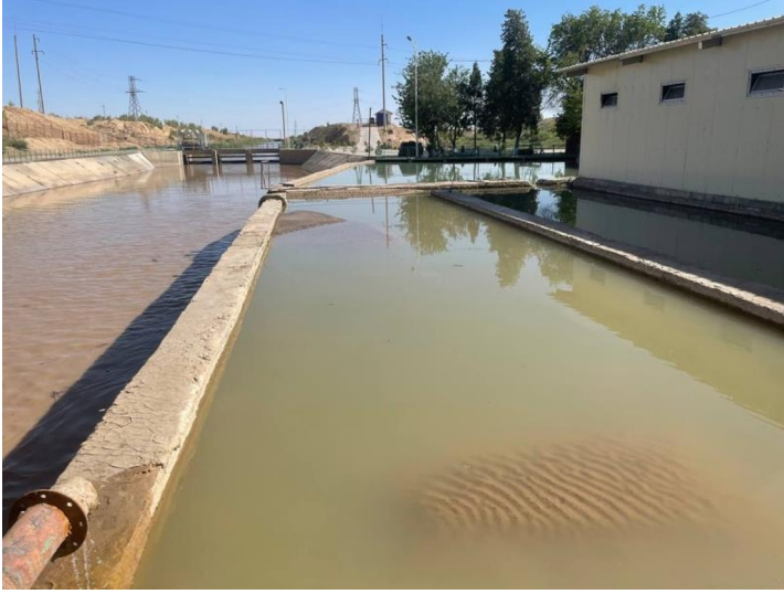
Fig. 6. Settling tanks for technical water of PS Kiziltepa.
