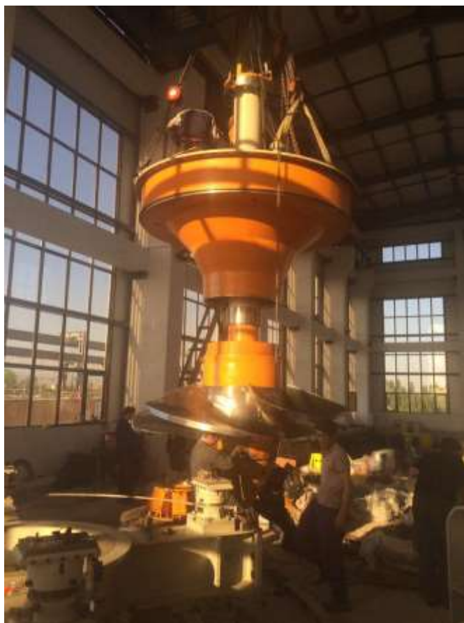
8.84-rasm. Mashina zalida burama kurakli turbinani o'rnatish
