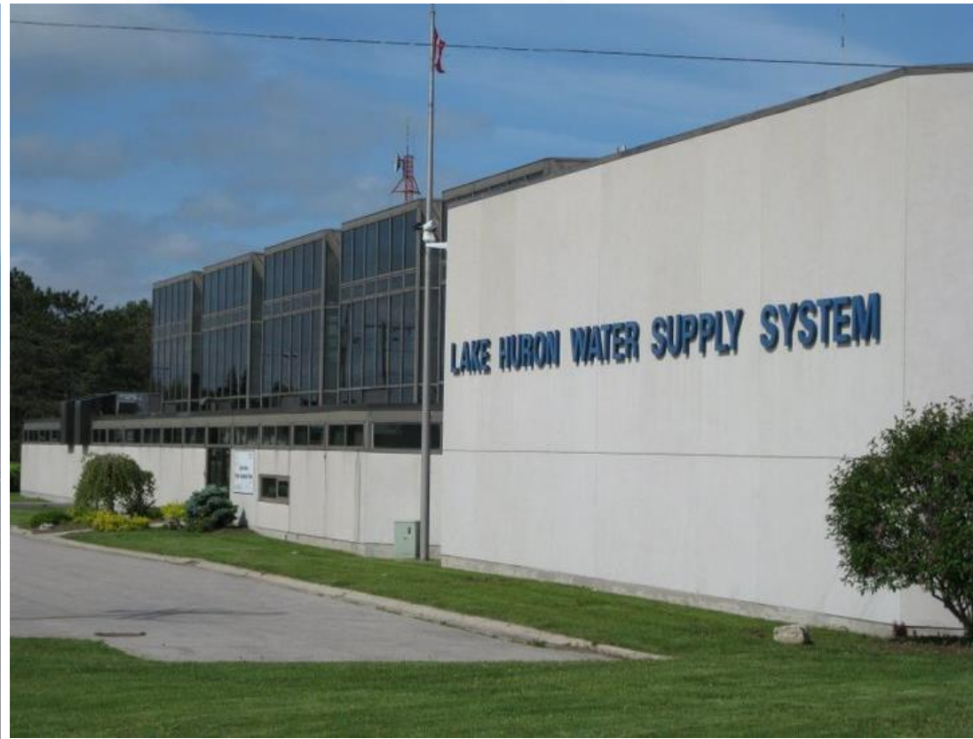
The lake water from Lake Huron is fully treated within this building before starting its journey to London.
