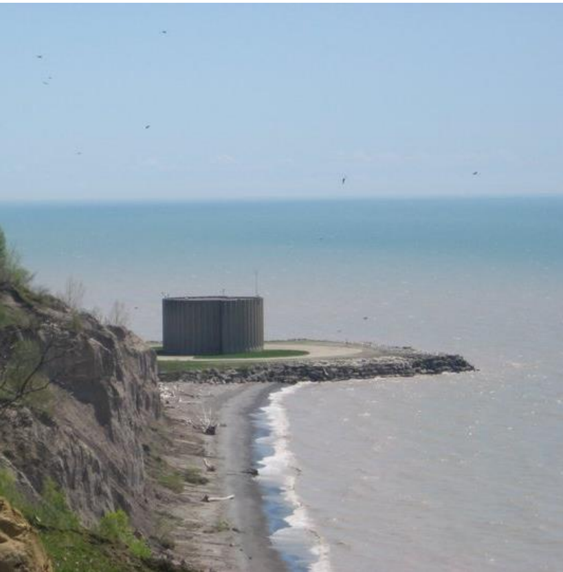
This is the low lift pump station which pumps the lake water from Lake Erie to the treatment plant.
