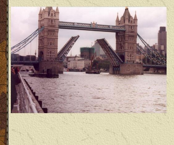
Tower Bridge is a bascule-bridge. The bascules will open to let ships pass through.
