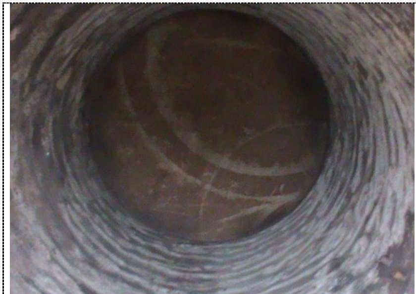
Figure 1. DN1420 mm pipe before shotcreting
