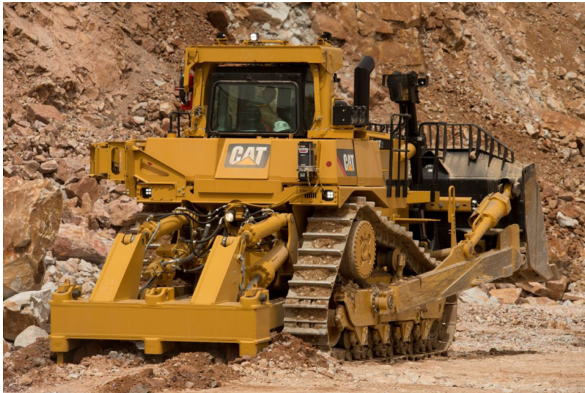
1-rasm. Caterpillar D10T2 Buldozer-yumshatgichining gruntga ishlov berish jarayoni.
