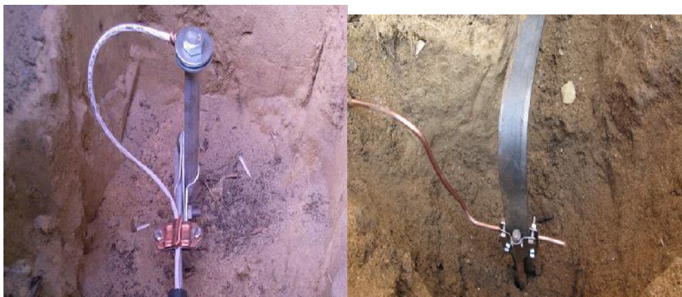
3.9 – rasm. Vertikal elektrodni transheyaga o'rnatish qurilmasi
