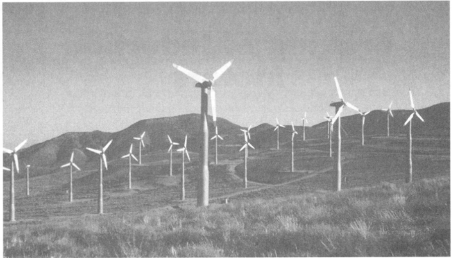
FIGURE 10.1 Photo of a wind farm located near Los Angeles, California
