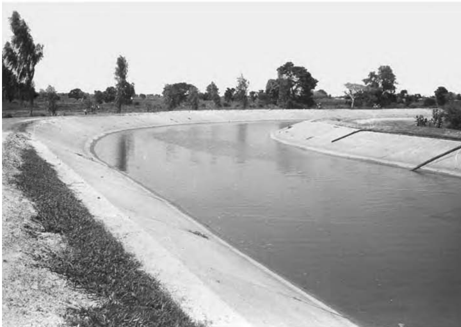
(b) A lined irrigation canal in Nigeria
