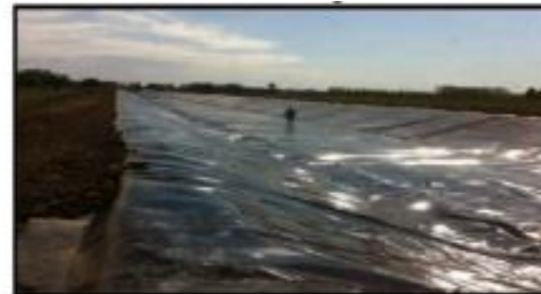
Fig. 2.2. – Geosynthetic membrane-lined irrigation canal
