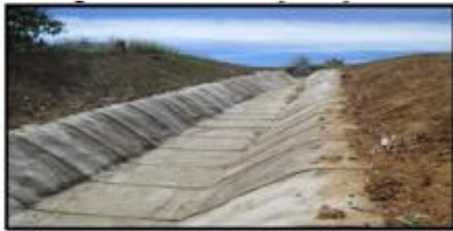
Fig. 2.1. – Concrete canvas-lined irrigation canal
