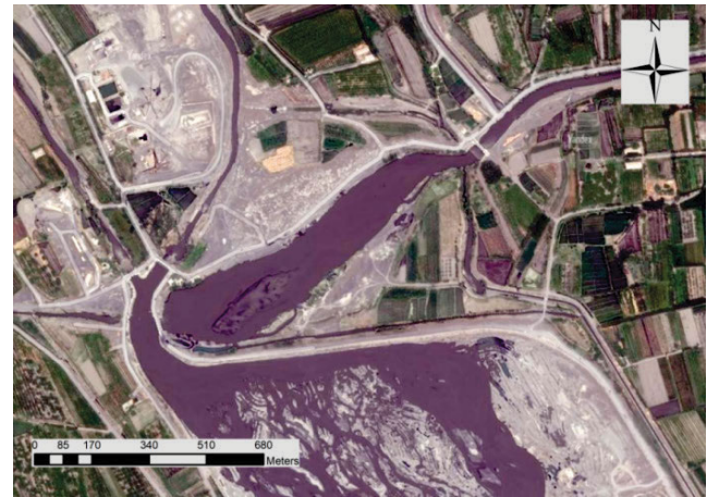
Fig. 1. Spatial image of the Kokand hydrocomplex; source: own elaboration
