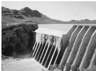
(e) Typical concrete dam
