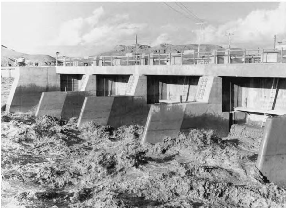
(b) Sluice gates controlling discharge into irrigation canal, Iraq
