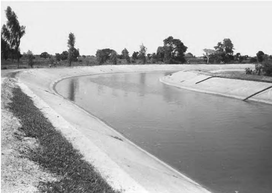
(b) A lined irrigation canal in Nigeria
