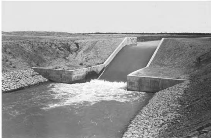
(b) Drop structure on an irrigation canal in Iraq
