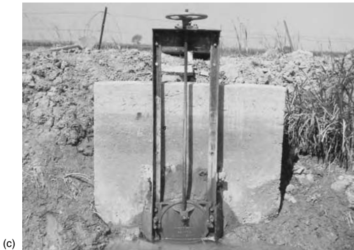
2.15 Forces on sluice gates.
