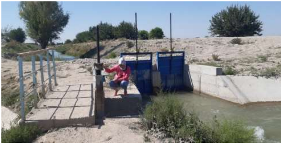
Figure 6. Studies at the sluice gate of the Sangrau Canal
