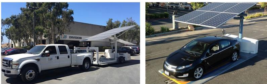
2.8 – rasm. Quyosh panellari bilan butlangan mobil zaryadlash stansiyalari
