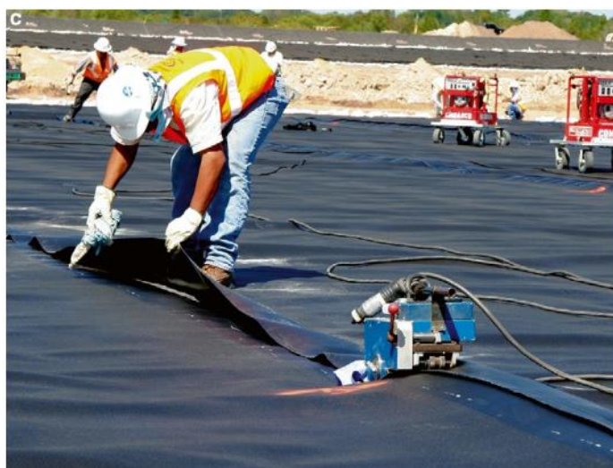
4.6-rasm Chiqindixona tagida himoya pardasini qurish
