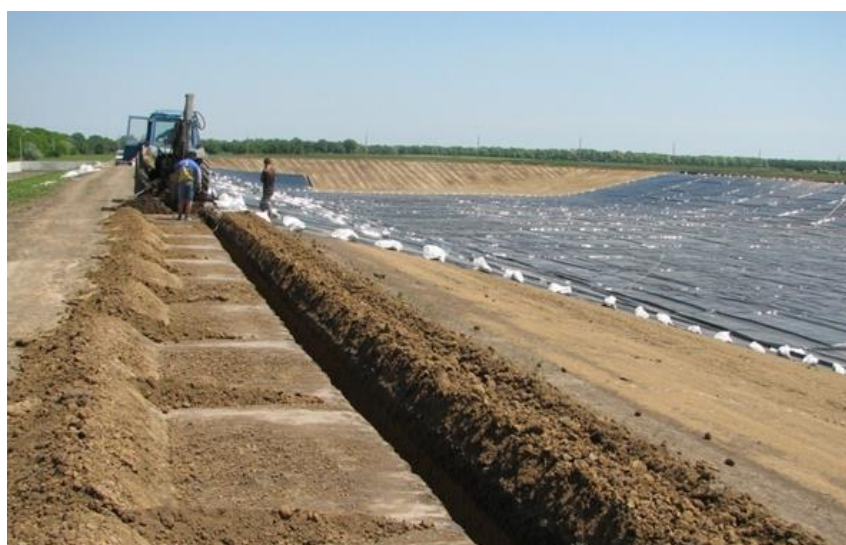
4.16-rasm - Gidroizolyatsiya materialini mahkamlash uchun ankraj xandaqi
