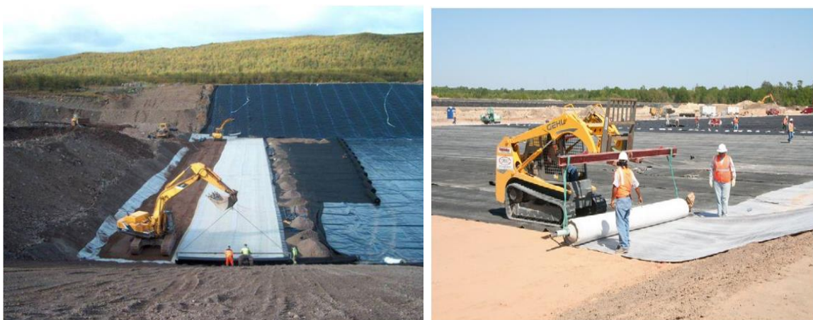
4.5-rasm Poligon poydevori uchun himoya moslamasi
