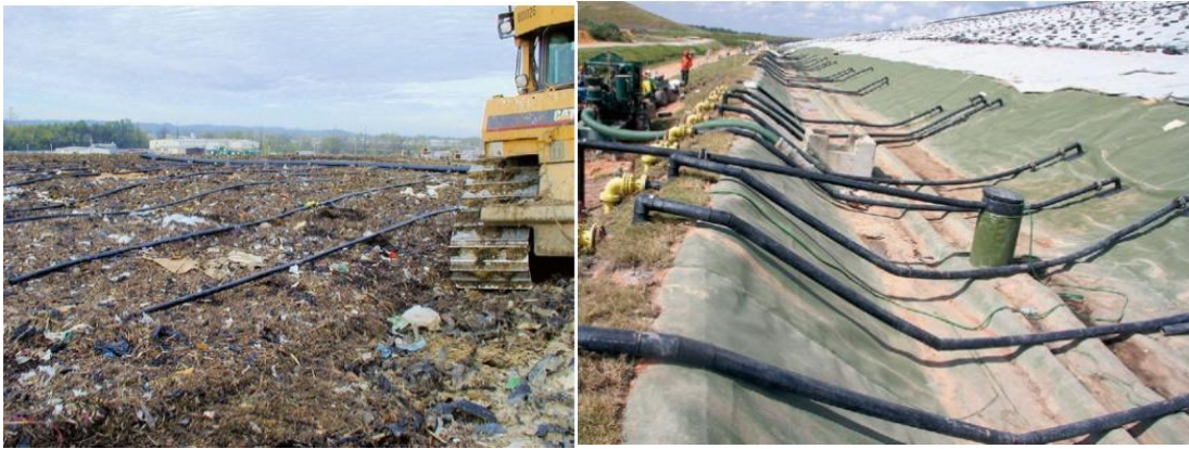
6.5-rasm Filtratni yig'ish tizimi
