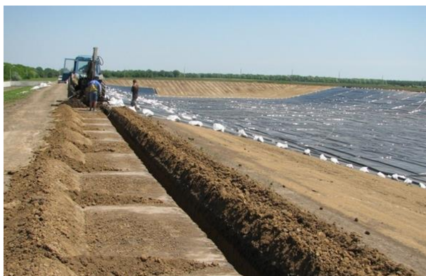
4.16-rasm - Gidroizolyatsiya materialini mahkamlash uchun ankraj xandaqi
