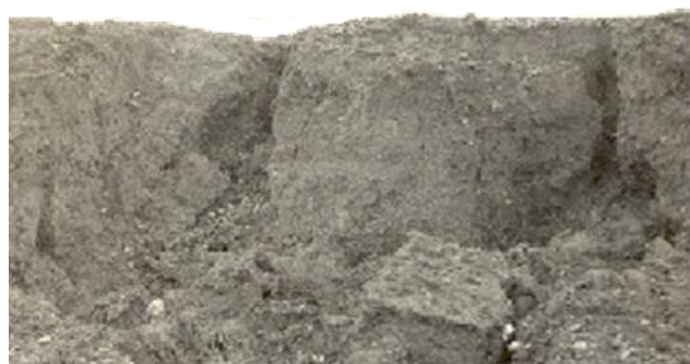
3.7.3-rasm. Sug'orish kanali ko'tarmasining yuvilishi jarayoni.
