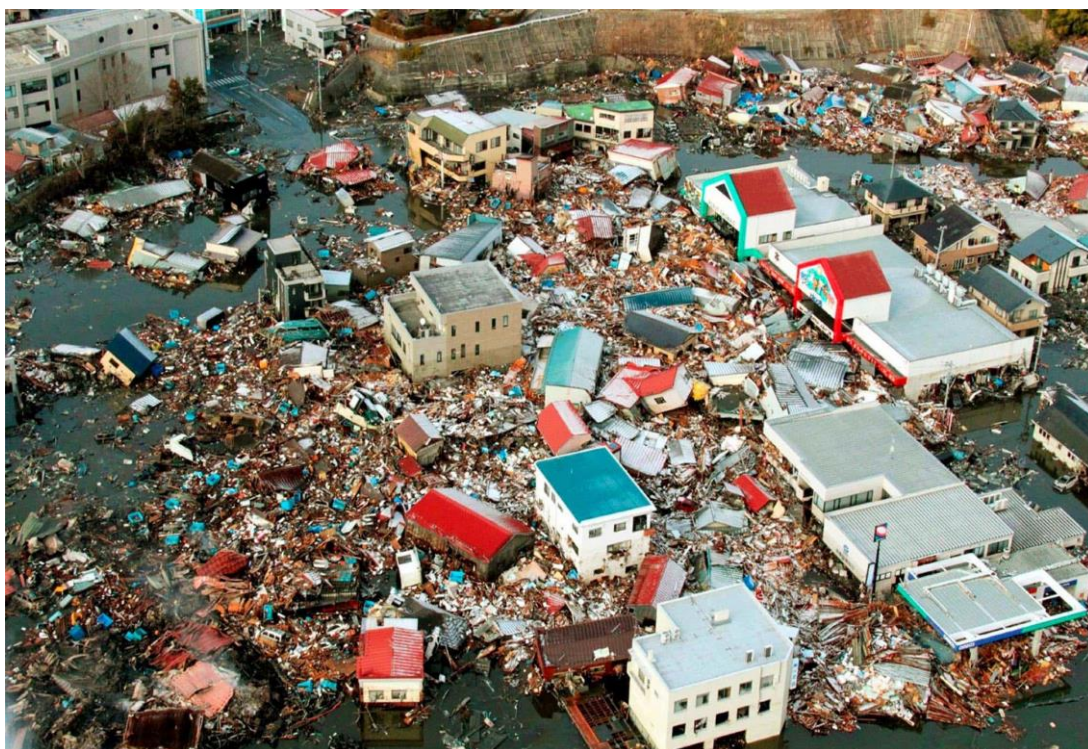
8.8-rasm. Sunami oqibatlari. https://kipmu.ru.tsunami .
