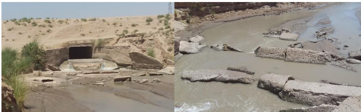
Picture 1.3. Deformation processes in the channel ducts of lower and middle water reservoirs (downstream channel Zang-9 in Surkhandarya region).
