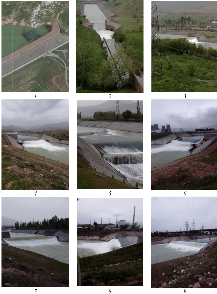
Fig. 3. Bypass channel with water-cutting energy absorbers of Angrenskaya mine 1) - water intake unit of the underground tunnel, 2) - a bypass tunnel with a dewatering energy absorber, 3) - the first water-breaking energy absorber, 4) - the second dewatering energy absorber, 5) - the third dewatering energy absorber, 6) - the fourth water-breaking energy absorber, 7) - the fifth water-breaking energy absorber, 8) - the sixth water-breaking energy absorber, 9) - the eighth water-breaking energy absorber
