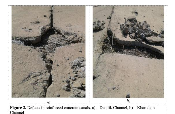
When analyzing the defects in Figure 2 above, we found that cracks and debris of different sizes in reinforced concrete slabs were mainly observed in areas where the water level in the canal varies.
