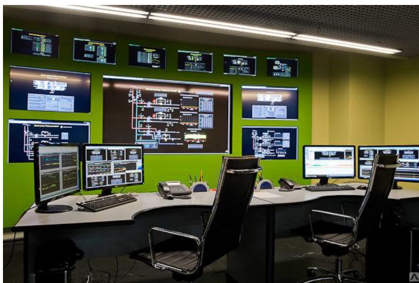
4.27-rasm. Suv ta'minotida dispatcherlik punkti bosh shit paneli
