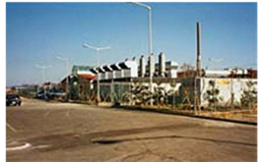
6,5 MW CHP in Seoul/South Korea
