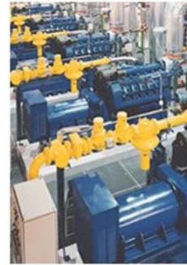
stationary CHPs in Mechernich 6x600 kW el
