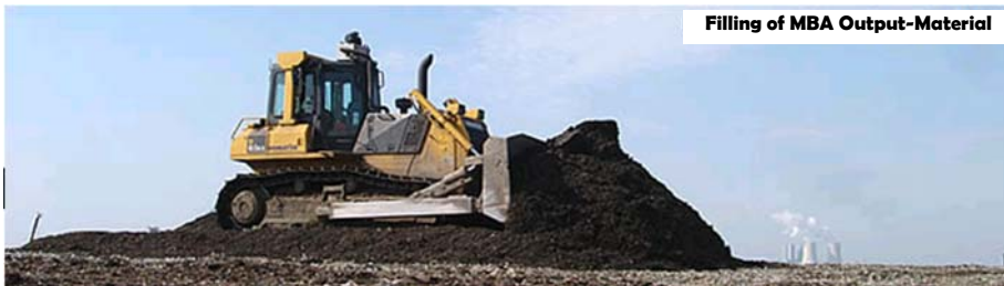
Intermediate cover after max. 2m
