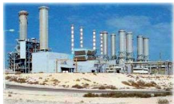
Jebel Ali Desalination Station, Dubai Lahmeyer International
