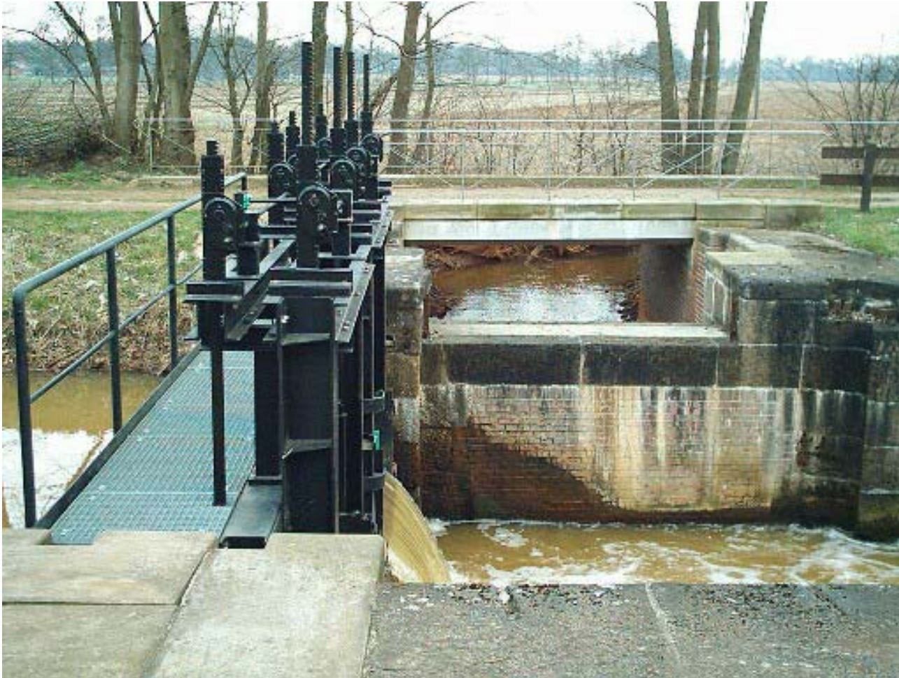
Weir with deduction building (Lohner Bach; Emsland)
