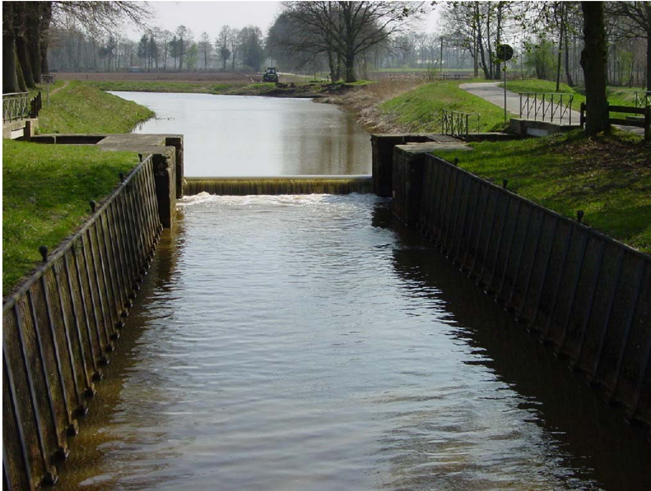
Fixation of embankment with cement and steelwall (artificial cataract)
