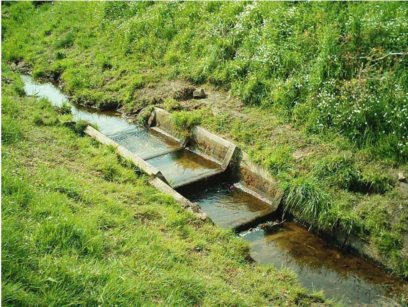
Fixation of the riverbed by cement basins (Lengericher Dorfbach/Emsland)
