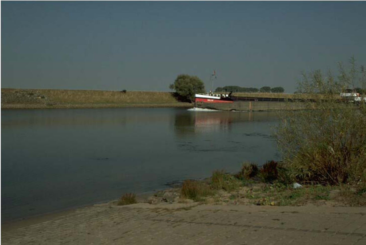
Cargo ship on River Weser. Banks with levee, moulded quarrystone rubble and paved ferryboat ramp
