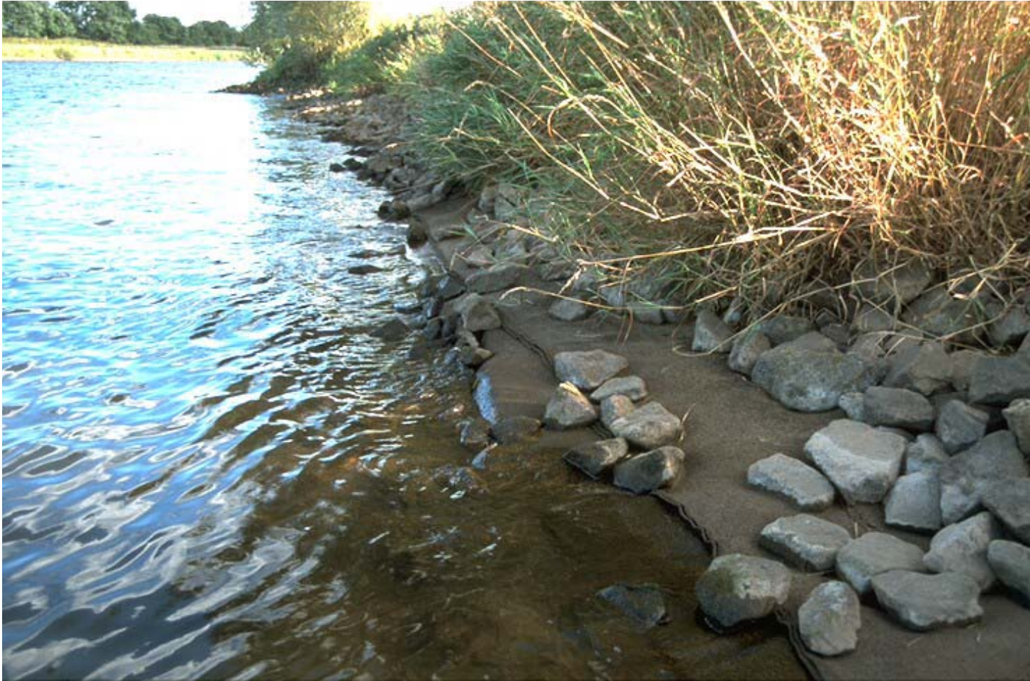
Fixation of embankment by quarrystone rubble and geotextile (Aller)
