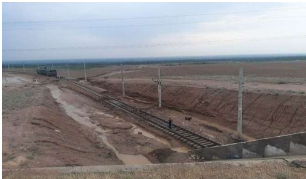
Figure 1. Impact of strong mudflows on the railway (Angren-Papal direction of the railway)
