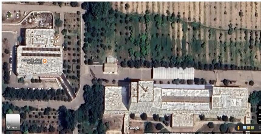
Figure 1. Top view of the 30 kW power plant installed in building 3 of the Institute.
