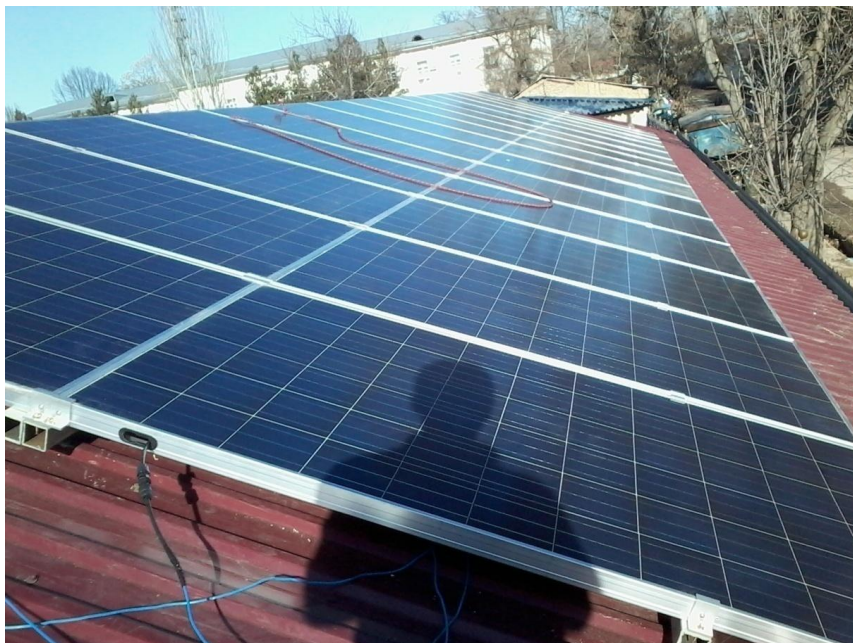
Figure 7. PVPs of the academic PV power plant installed at TIAME
