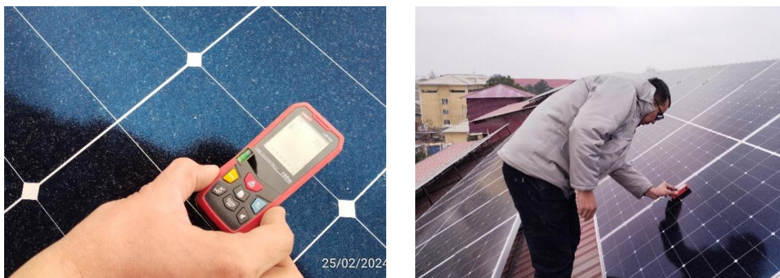
Fig. 6. The process of measuring solar panels horizontally in degrees
