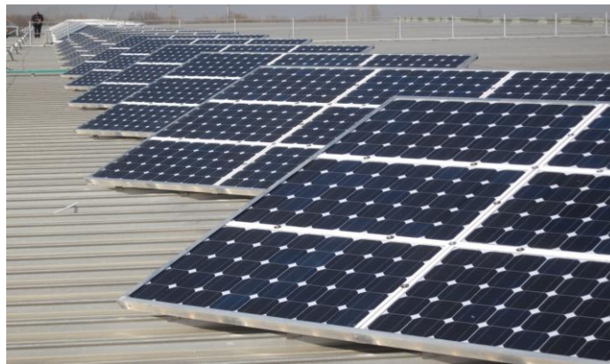
Figure 1. PVP with a capacity of 30kW installed at the Samarkand Cigarette Factory "UZBAT A. O." JSC JV
