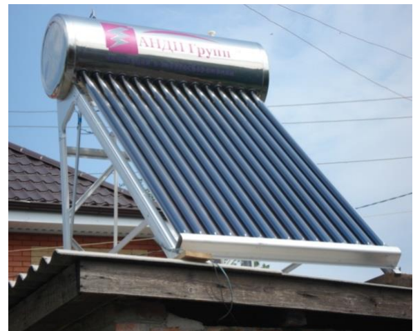
Fig 2.7. Installation of solar water heater collectors.
