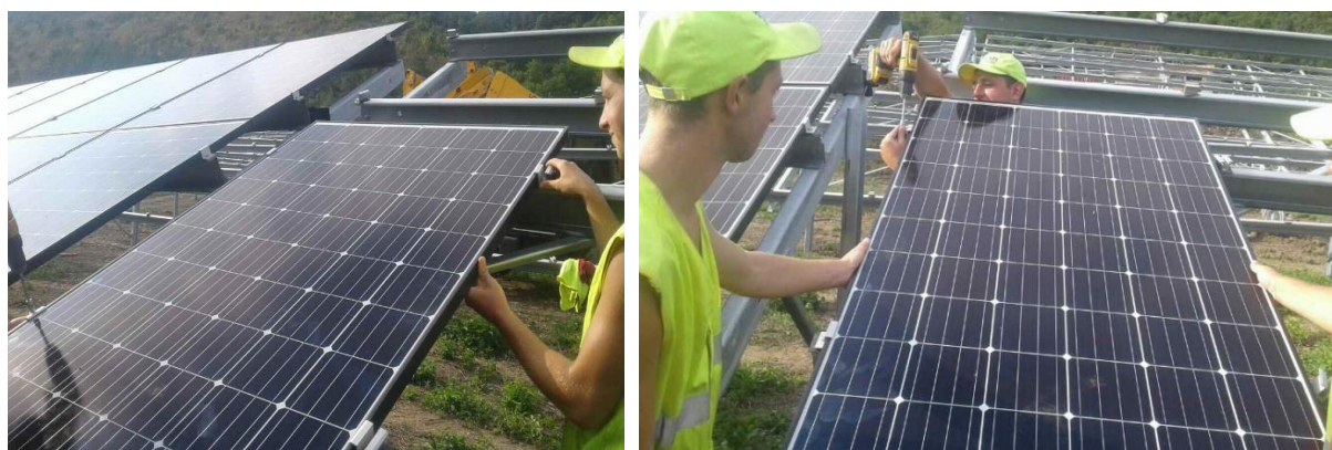
Figure 3.19. Installation of solar panels by engineers at a solar photovoltaic station
