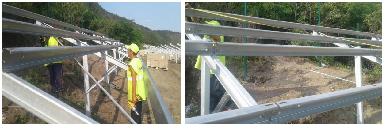
Figure 3.18. Installation of the frame part of the solar photovoltaic station
