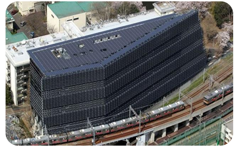
Solar panels installed in Japan
