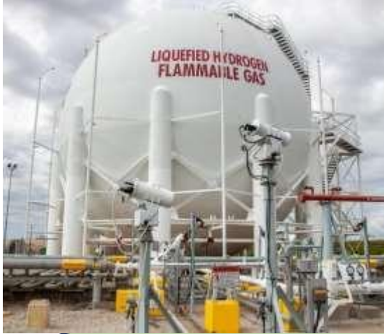
Liquid Hydrogen Tank at NASA's Kennedy Space Center since 1966
