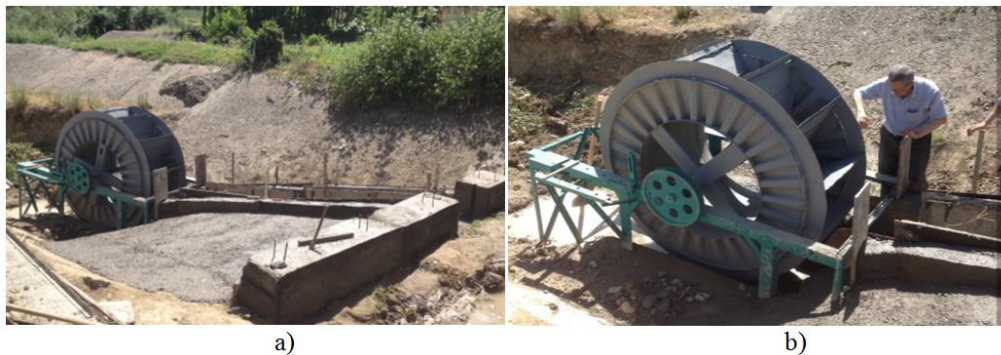
Figure 3. Installation of the device (a) and hydraulic structure (b)
