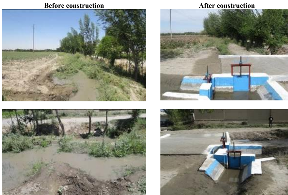
Figure 6. General view of “Asadbek” water distribution point (including the bridge)
