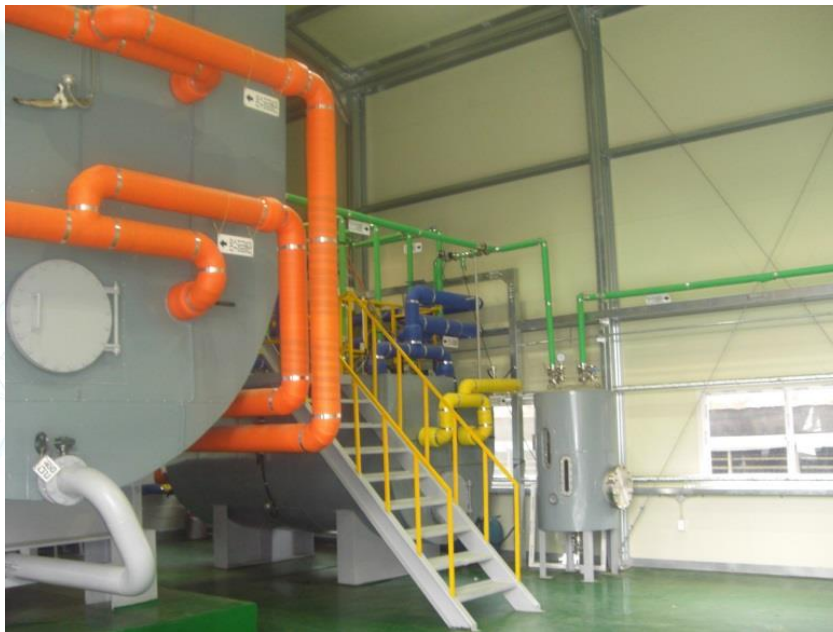
Picture1. Biogas device for processing organic waste from piggery
