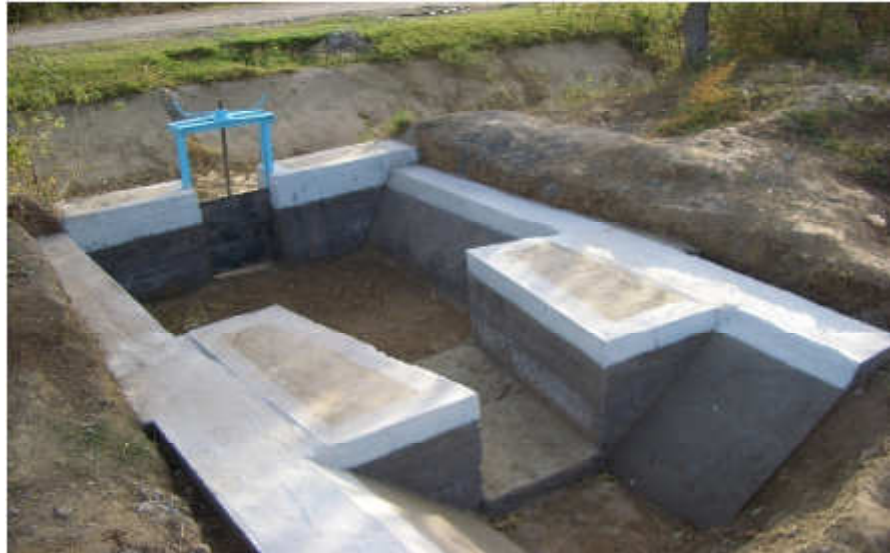
55-rasm. Suv o'lchash nasadkalari
