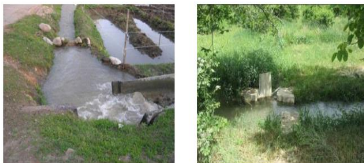
Figure 2. View of water measuring structure
