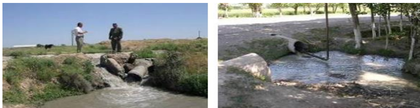
Figure 1. Condition of water distribution point
