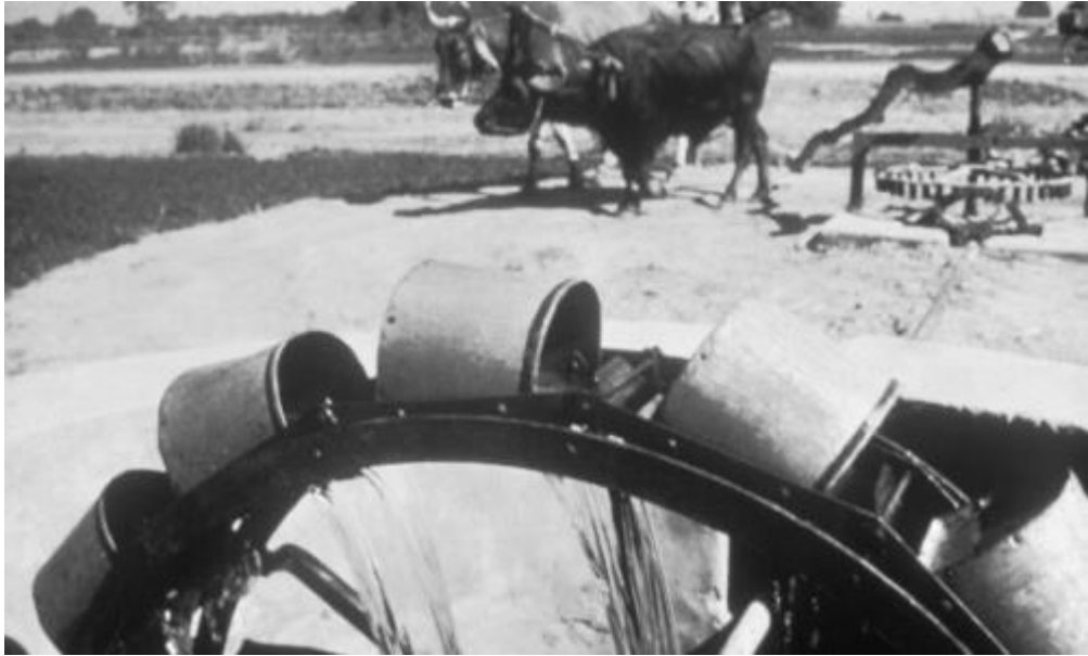
1.2-rasm. Xayvon kuchi bilan ishlaydigan chig'ir
