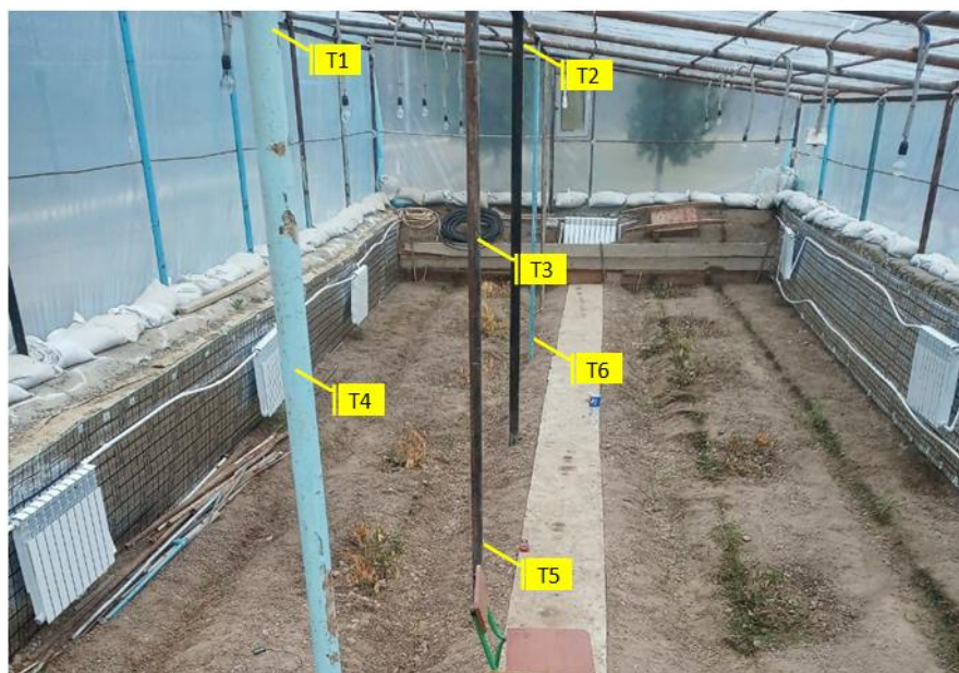
FIGURE 3. Installation of thermometers inside the solar-fuel greenhouse.
