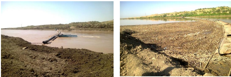
Fig.2. Inflow of bottom and suspended sediments in Karshi Main Canal
