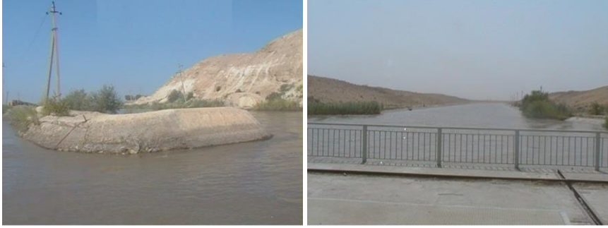
Fig.5. Destruction and siltation of sections of KMC canals "Compiled by the authors"
