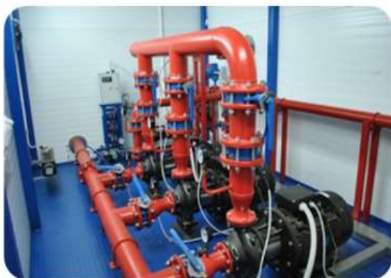
8.11 - rasm. Nasoslarning parallel ishlashi
