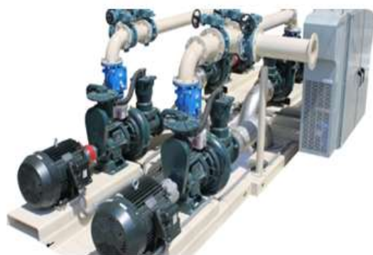
8.11 - rasm. Nasoslarning parallel ishlashi
