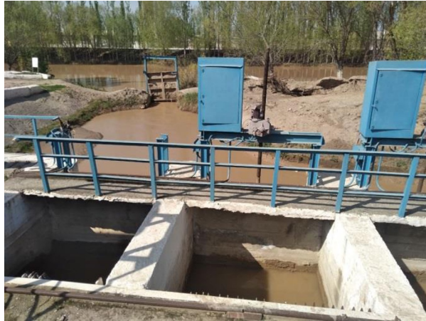
Fig. 2. Scheme of field experiments of BFC and SEC pumping station vanguard
